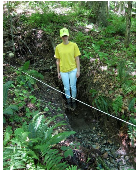
Jamie Dickhaus surveys erosion damage 2013.
