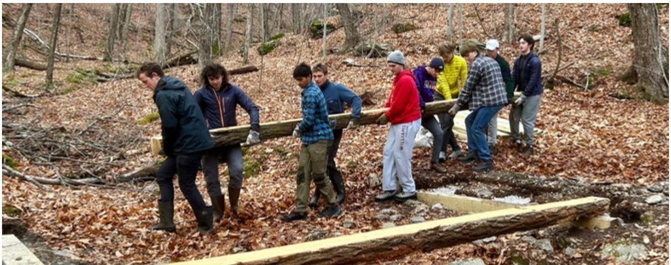
The men's crew team was instrumental in placing the large stream-spanning beams when rebuilding the bridge, November 2024.
